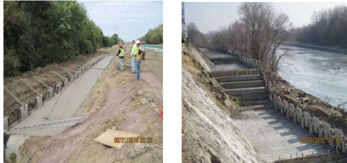
Plate (1-1): Application of lightweight foamed concrete fill in Sioux city, Iowa.
