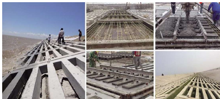
Plate (1-4) The use of GFRP in the sea walls in Yancheng city, China, 2016
