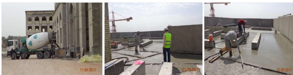
Plate (1-2): The use of LWFC in Al Hussain Quran School in Karbala city, Iraq, 2017.
