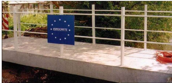
Plate (1-3): The first concrete footbridge in Europe reinforced with only FRP bars (ACI committee 440.1R, 2006).
