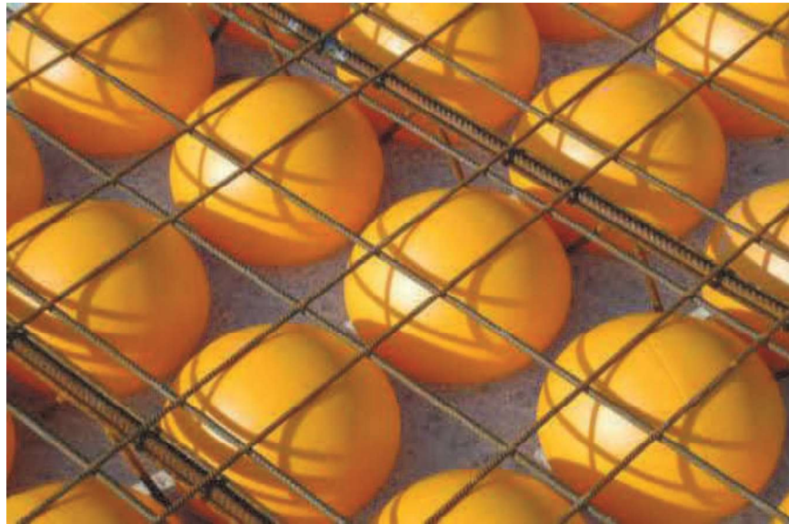
Plate (1-1) Bubble-Deck system (Bubble-deck, 2006)
