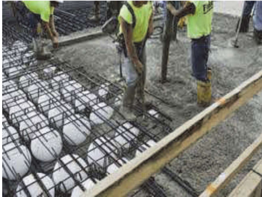
Plate (1-2) Construction of La Bahn hockey arena (Midkiff, 2013)
