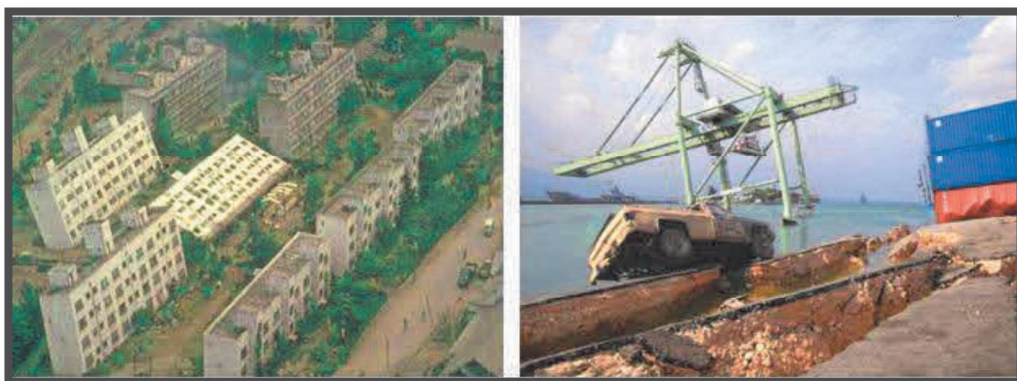
Plate 1.1 Failure of structure due to lateral load which result from earthquake
