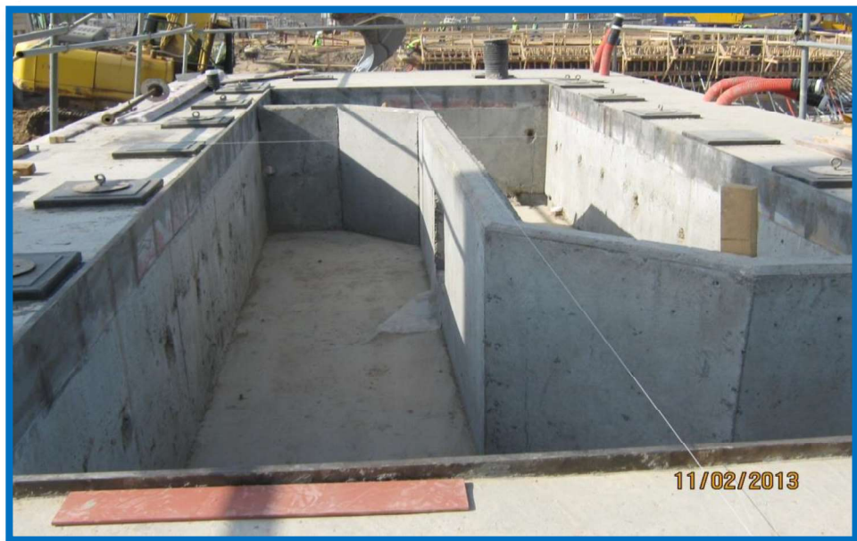
Plate (1.2): Turbine-generator foundation of Al-Mansuriya Station-Diyala/Iraq
