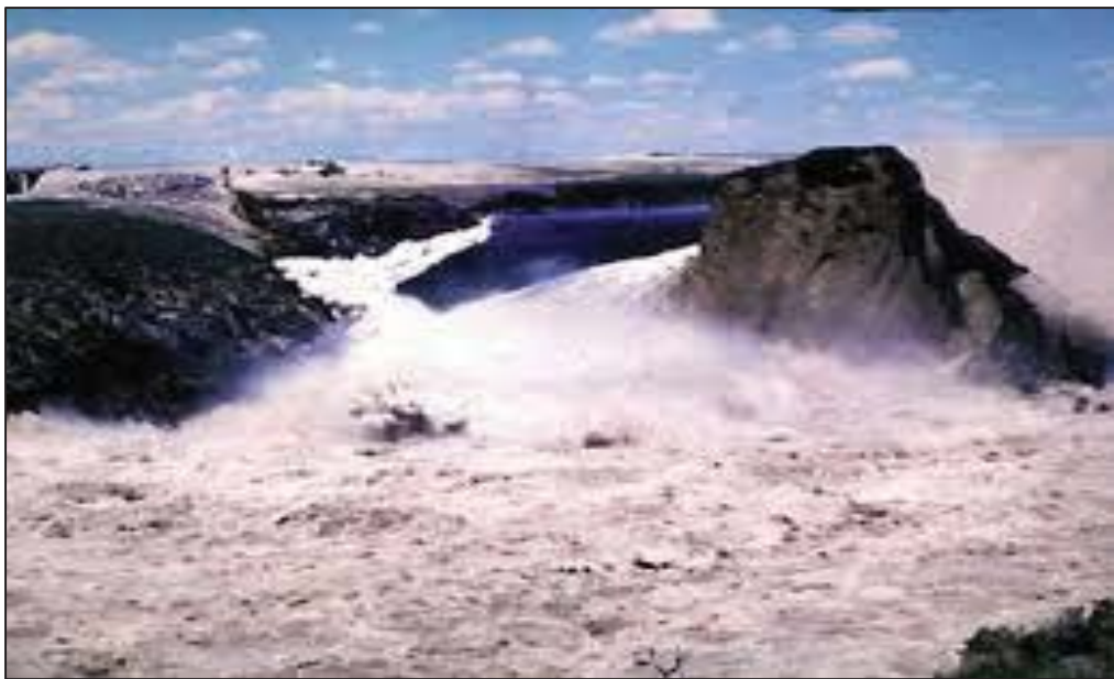
Figure 1.3 Teton earth dam collapsed(Perrow,1984)
