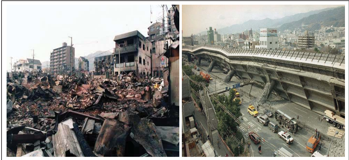
Figure (1.1) An example of damage caused by an earthquake (Kobe earthquake in 1995).
