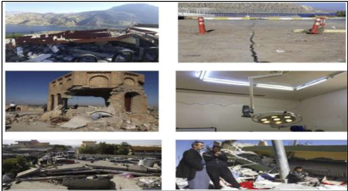
Figure (1.3): Damages to different structures in Iraq due to the Halabja earthquake, 2017 (after Al-Taie and Albusoda, 2019).
