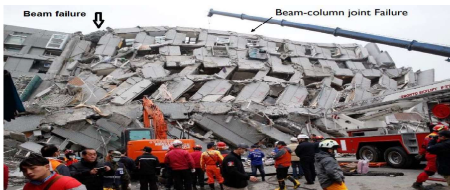
Figure (1-1): Collapse of the RC 6story building ( Shiohara, 2017 )
