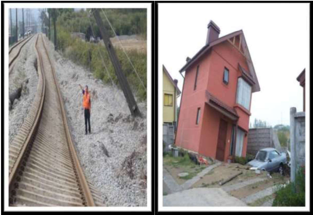
Figure 1-1 Liquefaction of flat areas. Condominium Brisas del Sol and railway near Concepción (Verdugo, 2011)
