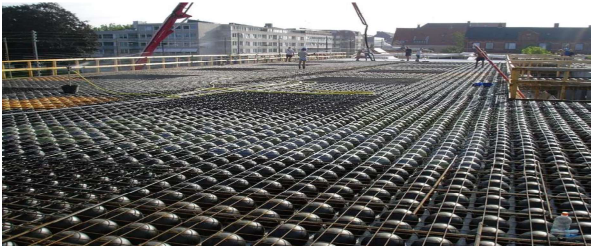
Plate (1-1) Bubbled RC Slab System ( www.BubbleDeck.com )
