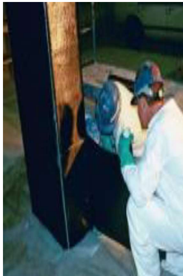
Figure (1-1): Jacketing of Columns by CFRP (Jijin and Prabhakaran, 2015)
