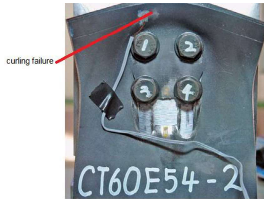
b. Curling failure, (Kima and Kuwamura , 2011)
