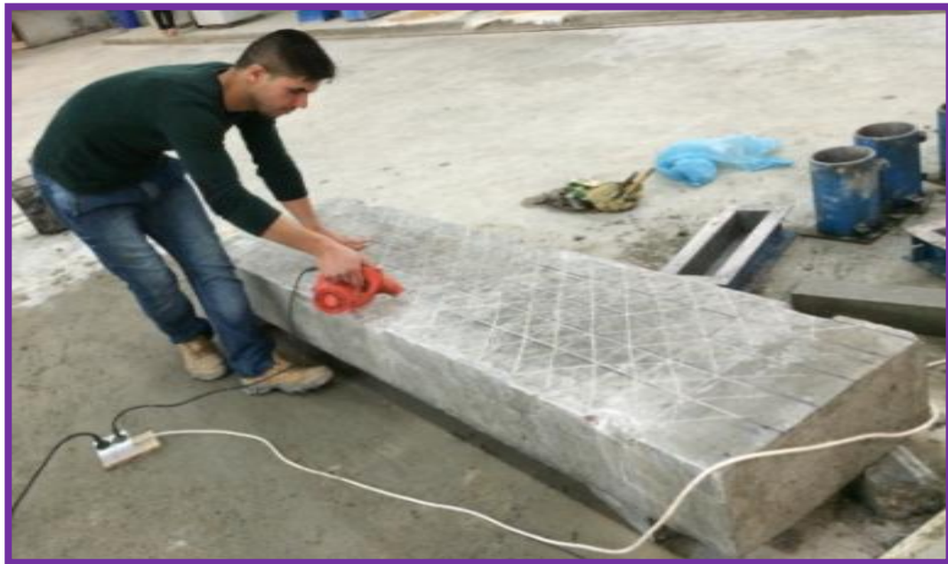
B- cleaning of surface
