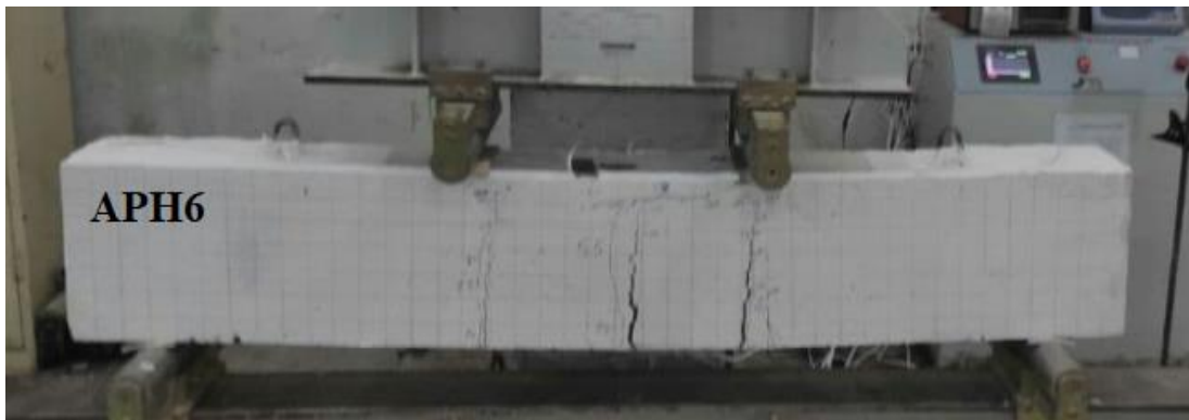
Figure 6. Crack pattern of APH6
